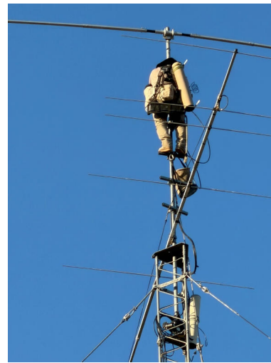
N6RO Tower Maintenance, Photo by Gary NA6O
